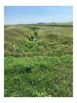
Outlet from Watonwan JD-11 with sloughing and instability and is an inadequate outlet for the project.
